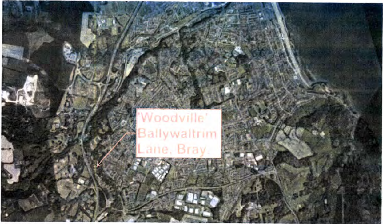
Aerial Image 1: The subject site is located on Ballywaltrim Lane, on the outskirts of Bray, Co. Wicklow.
